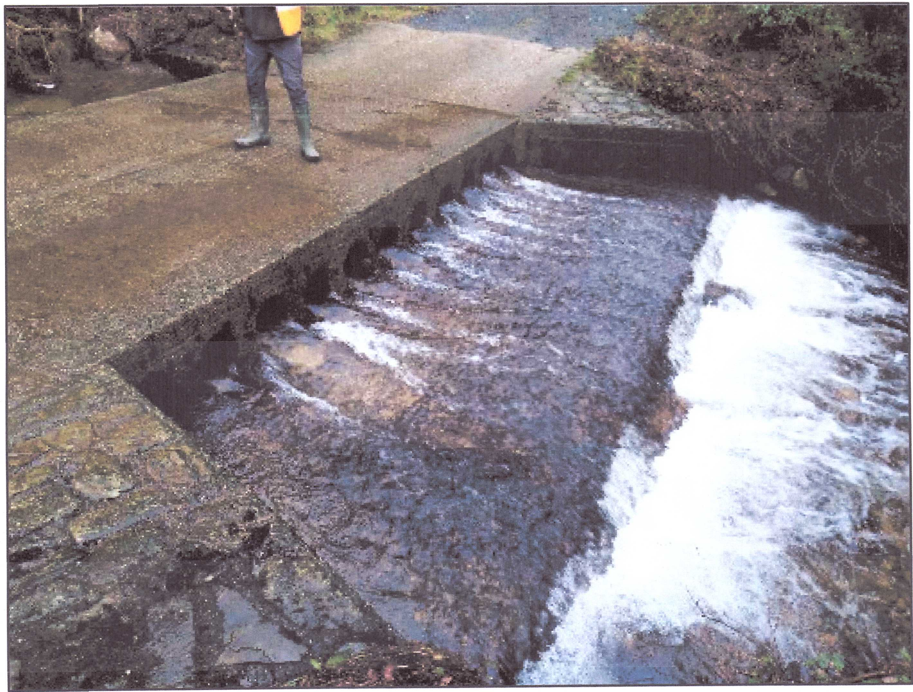
BALLYBOY BARRIER DOWNSTREAM VIEW
