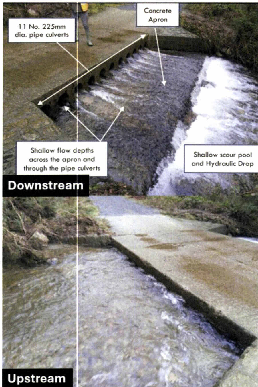
Figure 1-1 Ballyboy Culvert – Stantec (2026)
