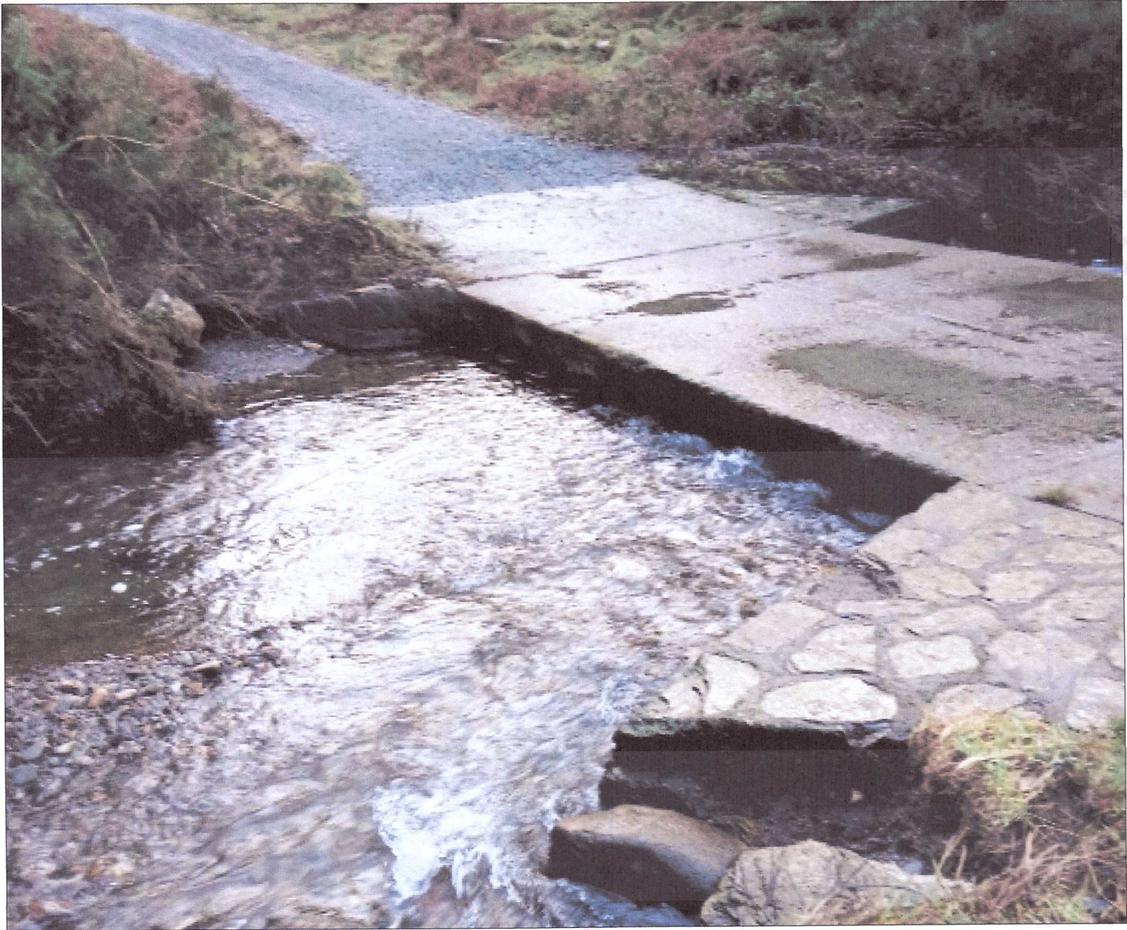
BALLYBOY BARRIER UPSTREAM VIEW
